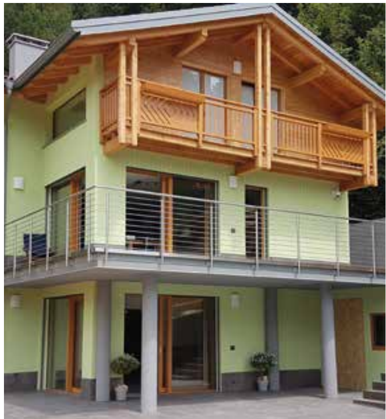
Detached house with timber frame System with eHPoca heat pump Ledro, Italy
