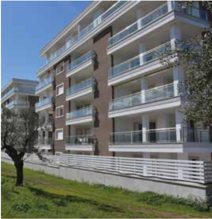
Next Village, 50 apartments Independent systems with 3in1 heat pumps Viterbo, Italy
