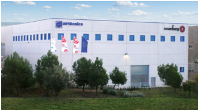
Airtècnics headquarters in Castellar del Vallès (Spain)
