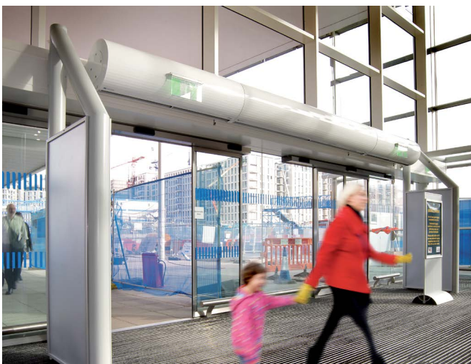
Rund Tailor made-linear installation for large openings
